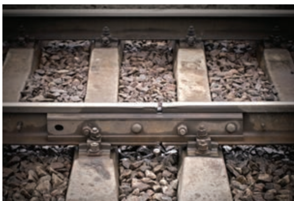
Figure 1.1 Gap in railway track
